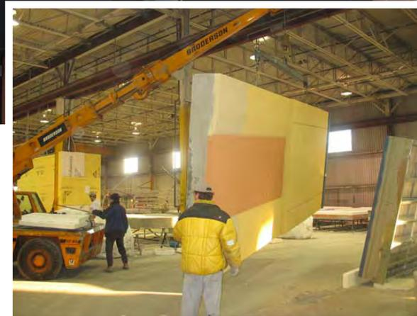
**An example of the prefabricated panels used by Lido Wall Systems to meet the project demands.**
